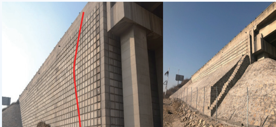
Special reinforcement and maintenance was carried out to reinforced retaining wall in specific section
