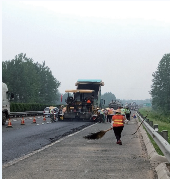
Preventive and reparative maintenance construction were carried out to roads
