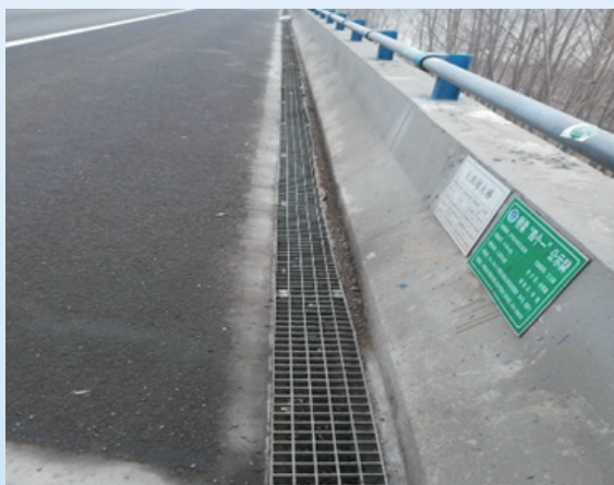
Renovation on rainwater channeling and drainage system
